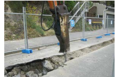
Trenching, pit building, ground excavation
